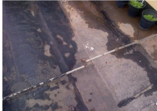
Plate 5: Broken water pipe.
