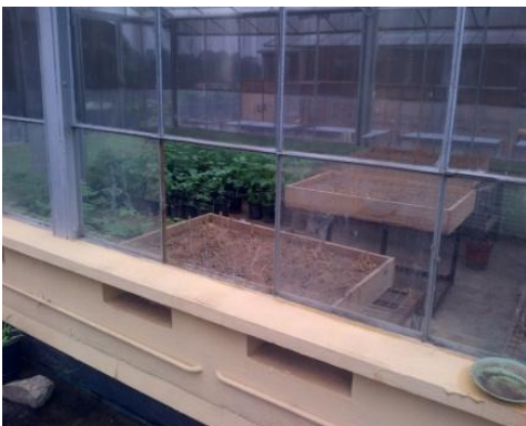
Plate 7: Glass section missing.
