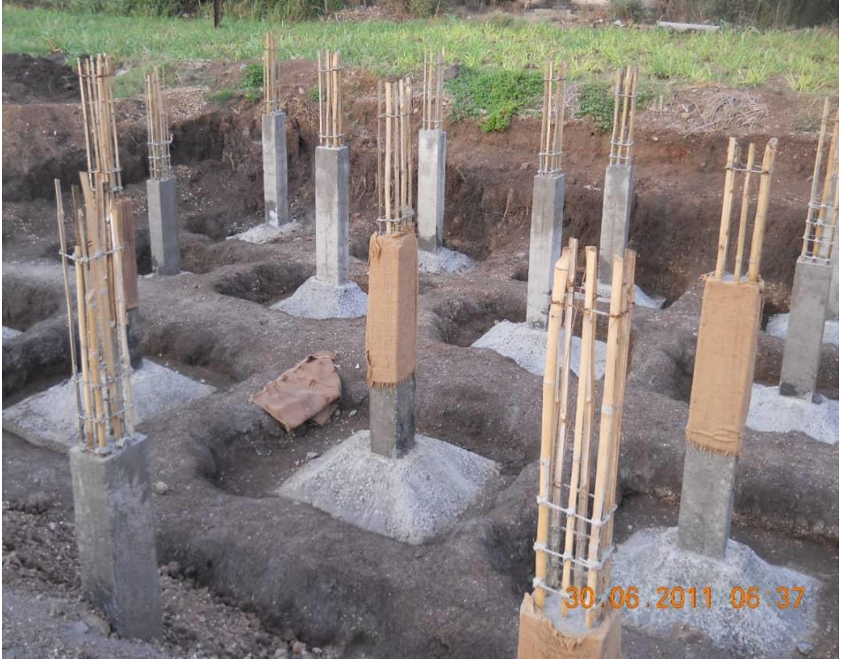
Figure 4: Bamboo as Reinforcement Material for Column
