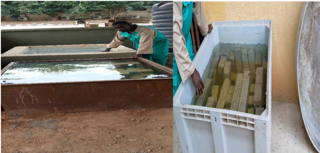
Figure 3.10: Curing in progress
