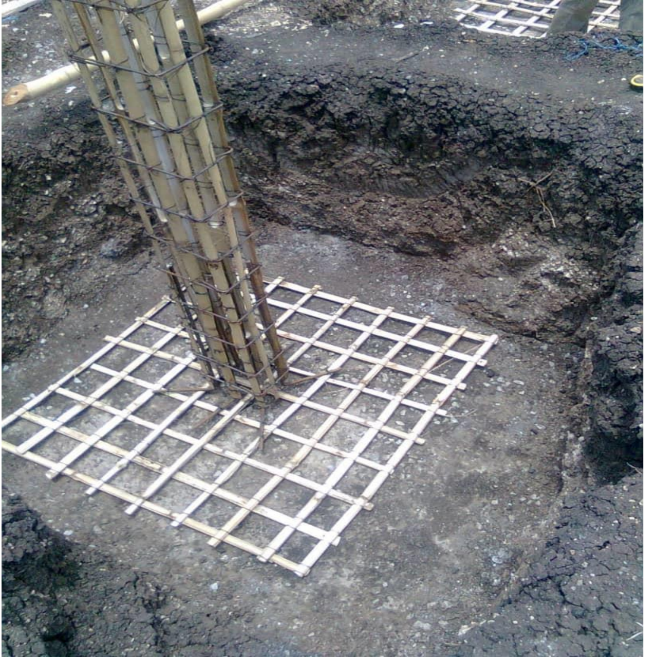
Figure 6: BR used for Column Starter Bar
