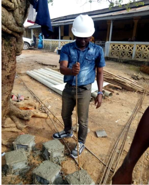
Plate I: Compacting of concrete in layers.
