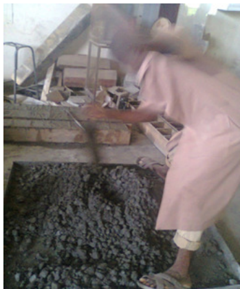
Plate III: Mixing of concrete
