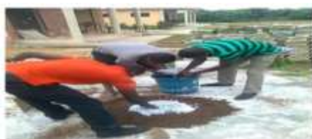
Mixing of paper, cement and sharp sand
